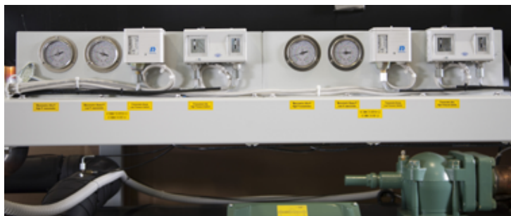
Manometri/pressostati refrigerante Refrigerant gauges/pressure switch
