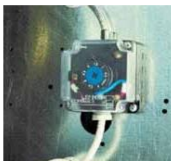
Pressostati differenziali aria Differential air pressure switches
