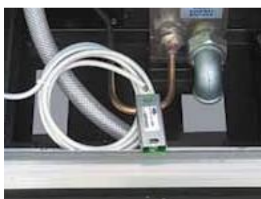
Sensore d'allagamento Water flooding sensor
